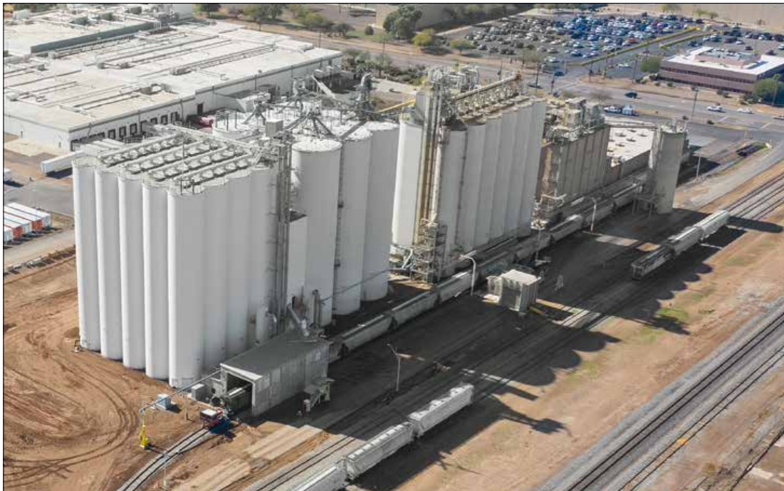
Aerial view of the Bay State Milling Company flour mill in Tolleson, AZ, with new 1-million-bushel elevator annex at far left. Photos courtesy of McCormick Construction Co.
