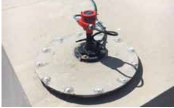
Radar can be mounted on flat or angled roofs and in segmented silos
